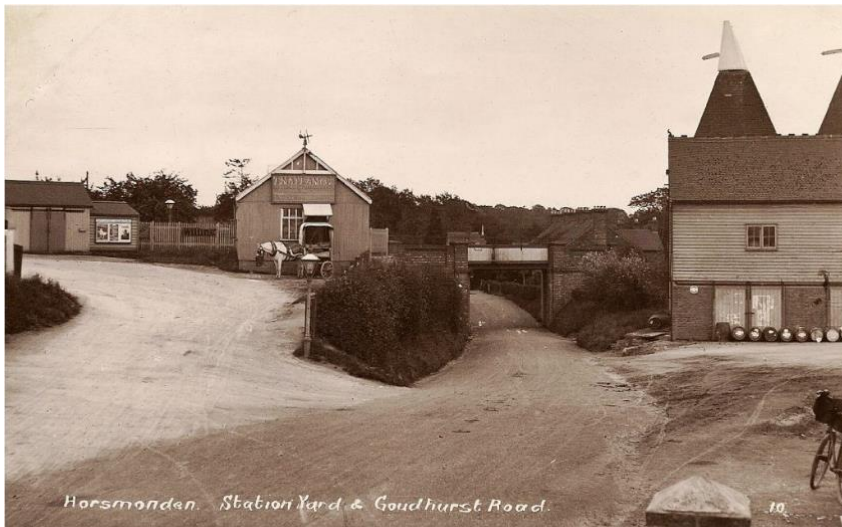
Plate 29: Historical Photo (date unknown) showing the railway bridge over Goudhurst Road. Bassetts Cottages would be just behind the bridge (Horsmonden Village Kent website).
