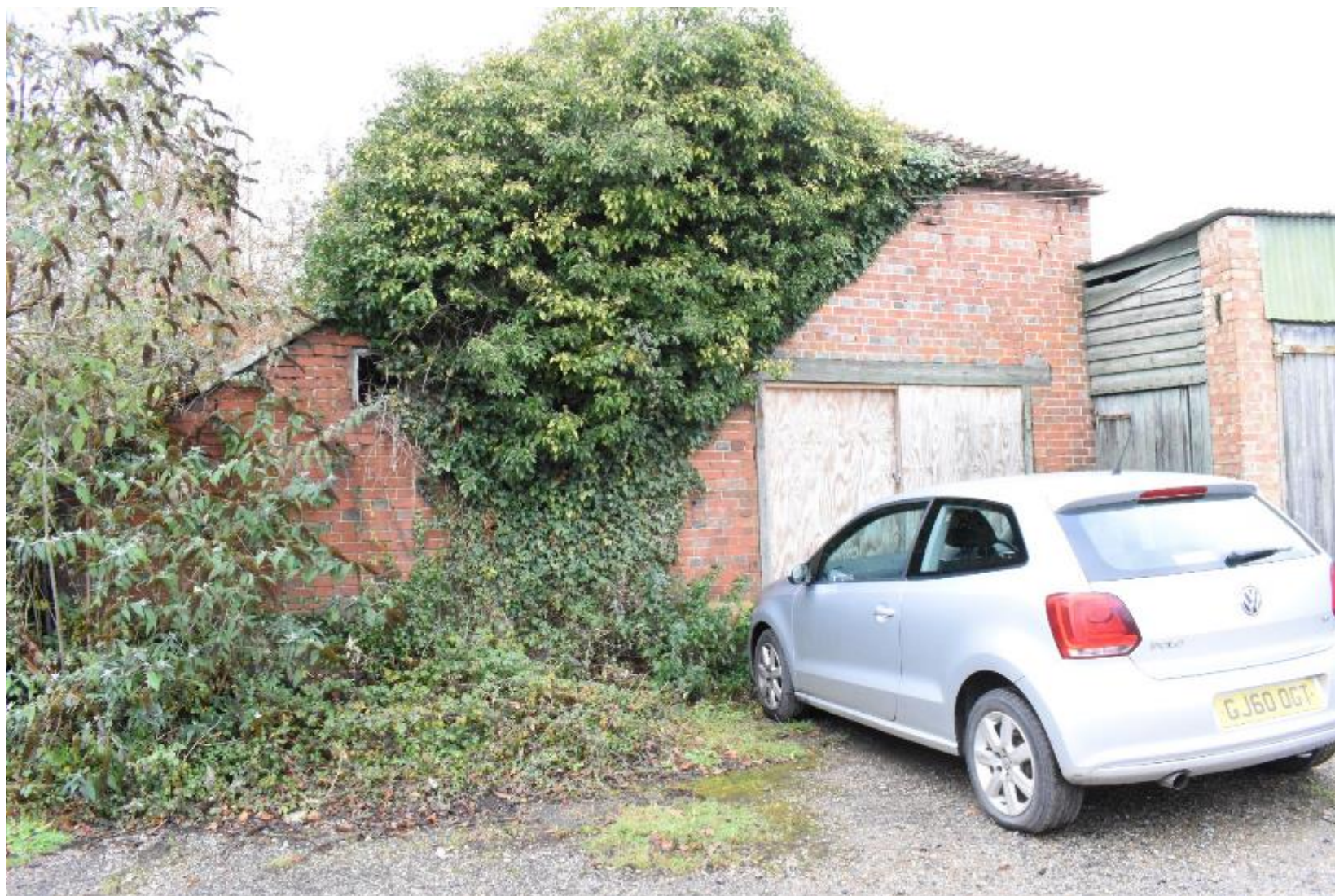
Plate 9: View of the potential 18 th century building (facing NW).
