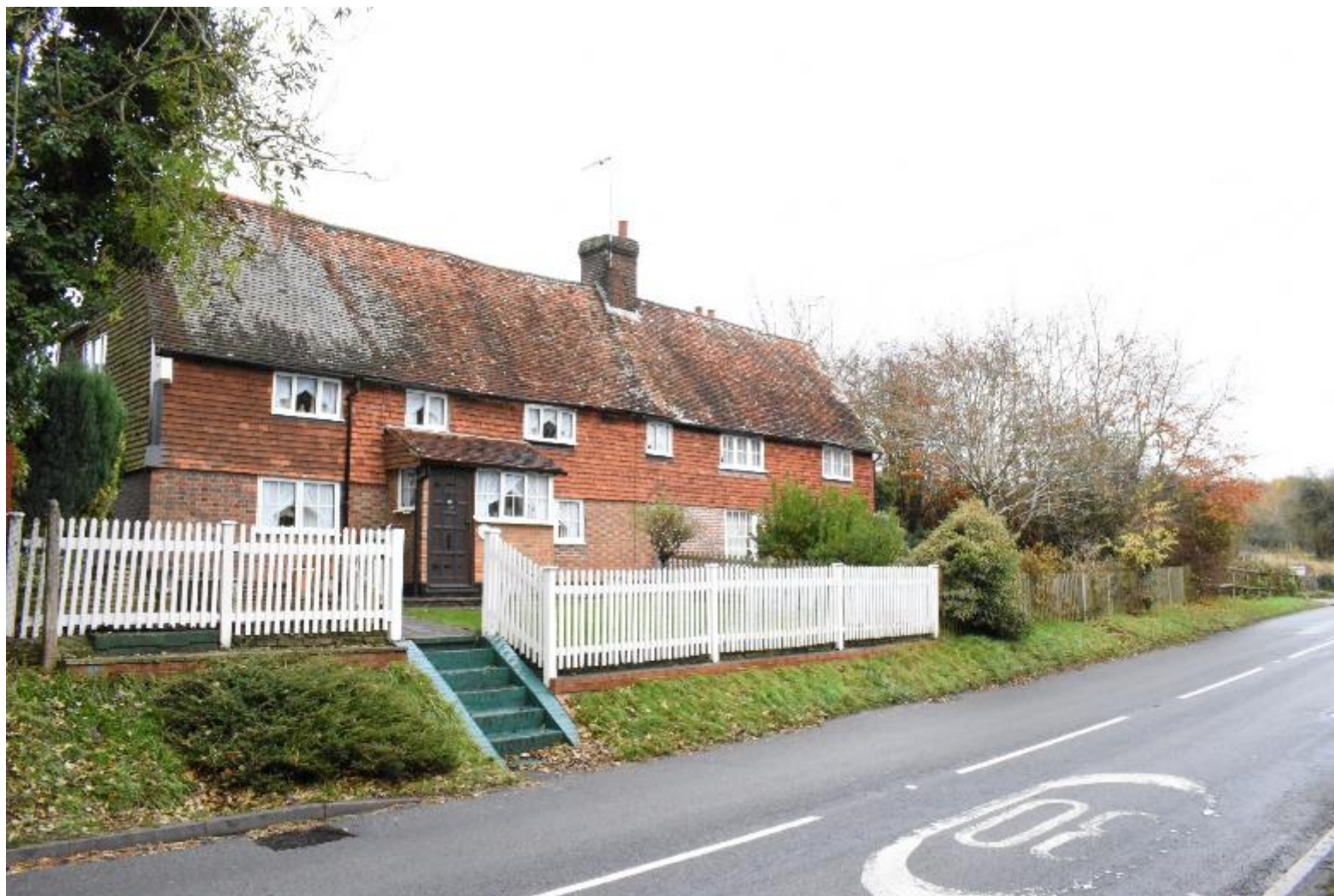
Plate 23: View of Old Bassetts Cottages from Goudhurst Road (facing NE)
